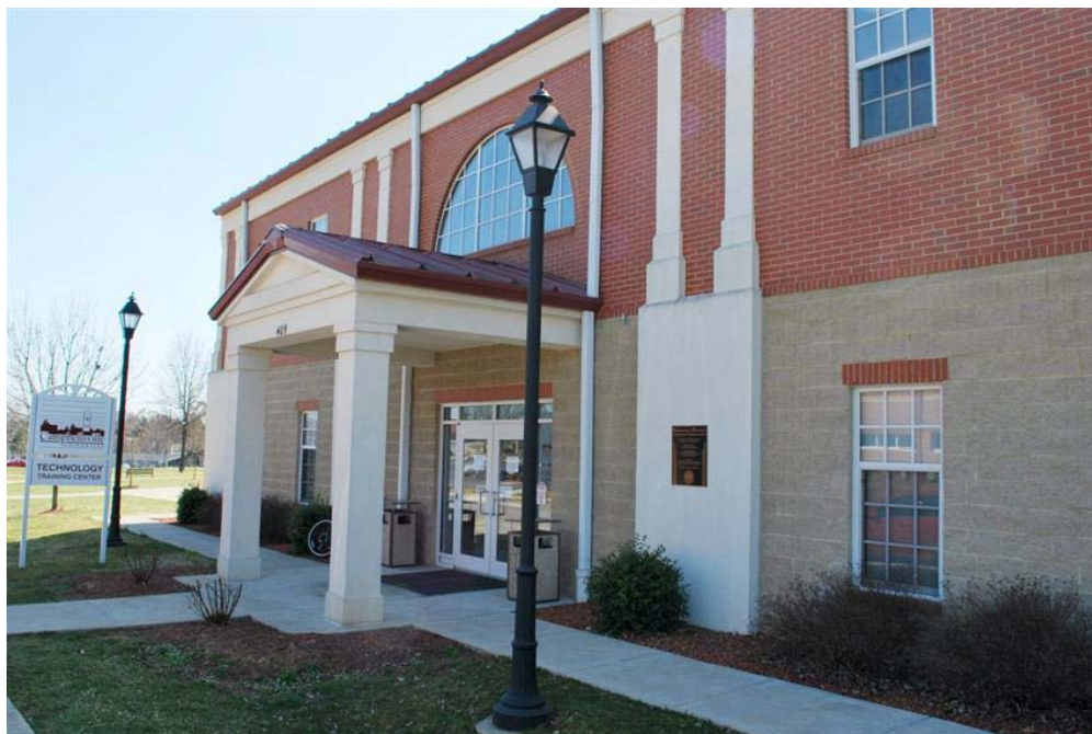
Technology Training Center (TTC), 409 North Hoskins Avenue, Campbellsville, KY 42718
